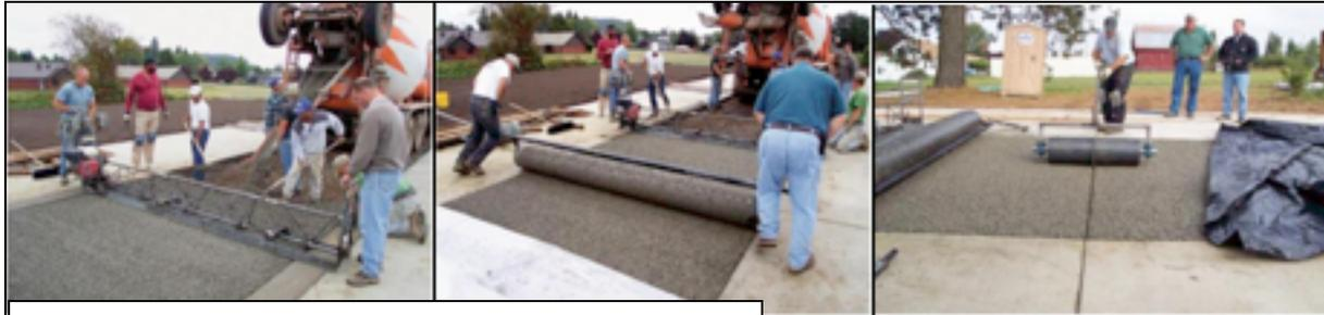
Figure 4: Sequence of Placing Pervious Concrete
