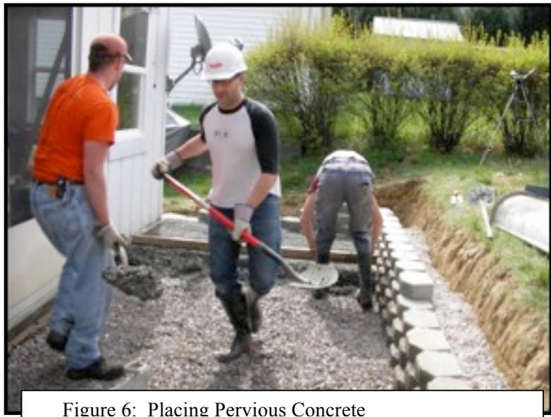
Figure 6: Placing Pervious Concrete
